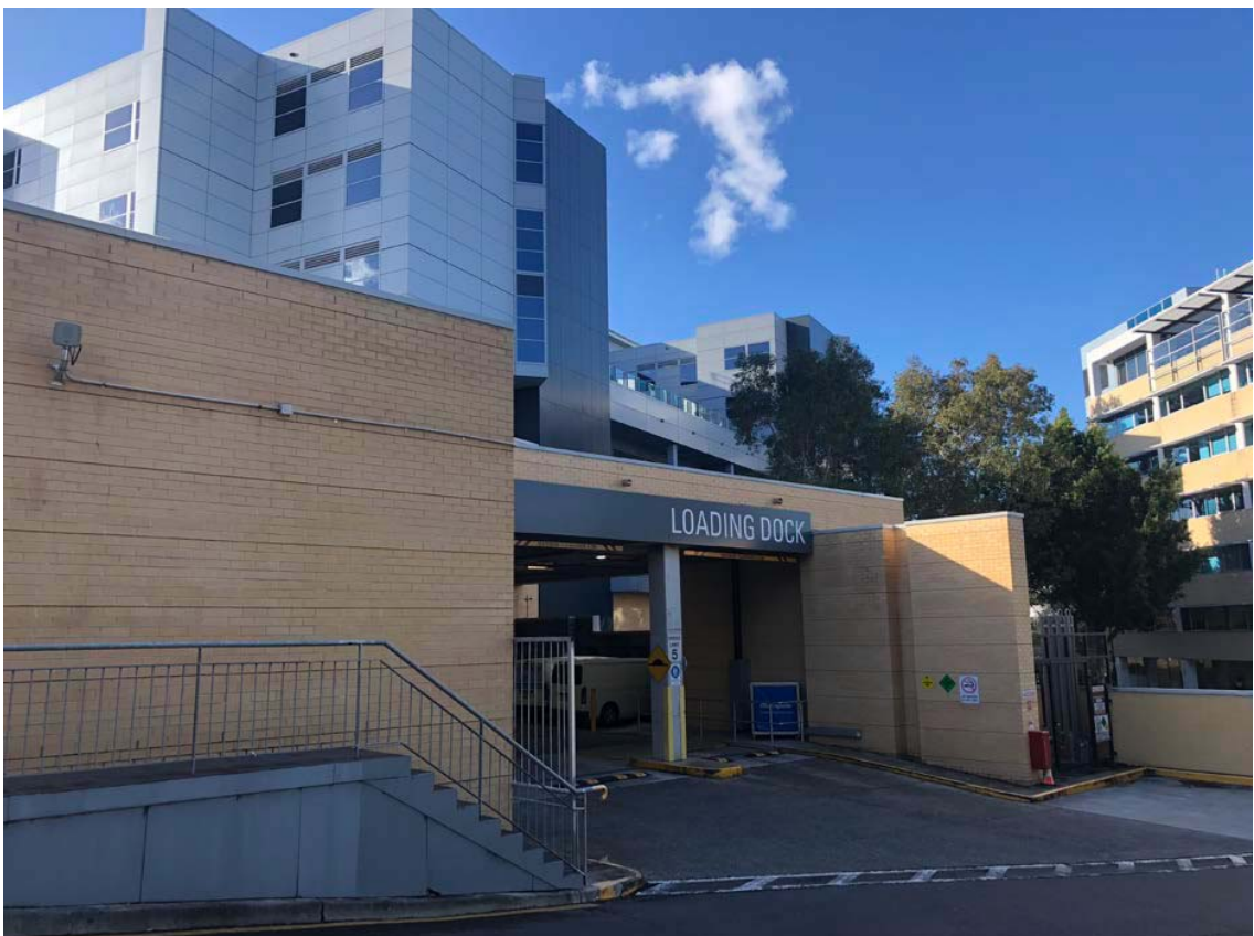
Figure 4: Macquarie University Hospital and loading dock adjoining the site.
